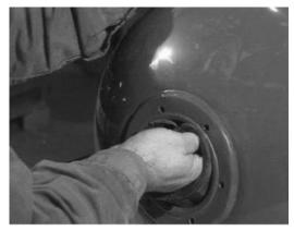
Avoid rubber on threaded holes, make the neck adhere to flange and centre the membrane
