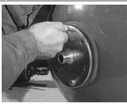
Replace the counterflange so that it presses the neck of the membrane against the flange ot the tank
